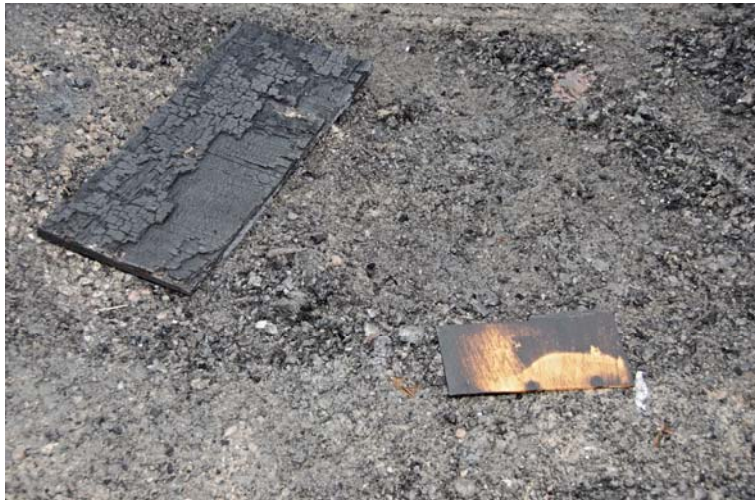
Figure 3: Charred panel from Test 18 showing fire degradation
